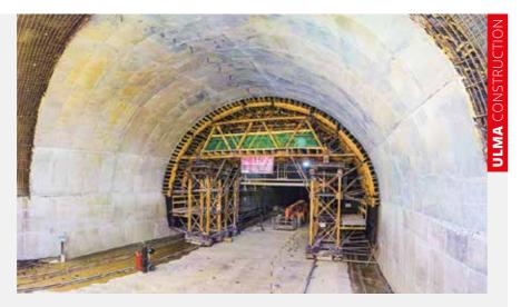
shuttering and pouring phases, lightweight COMAIN Handset Panel system was used to create the single-sided formwork necessary for the tunnel walls.
